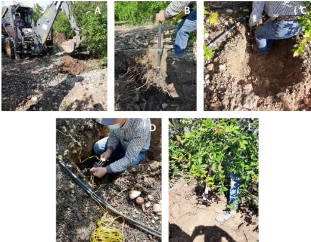
Figure 5. TDR Sensor Installation in a pomegranate farm
