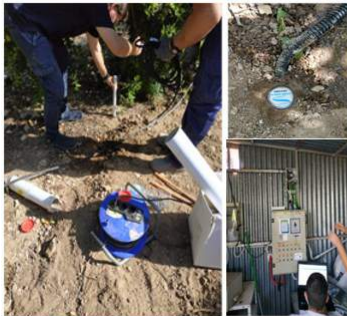
Figure 26. Instalation of the Drill and Drope soil probes.
