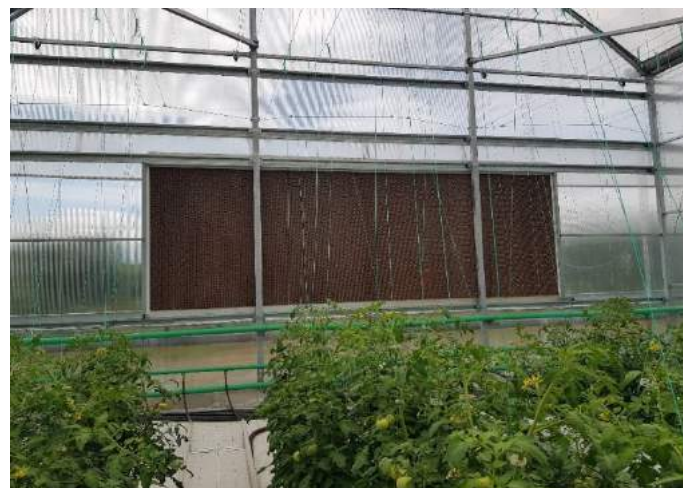
Figure 11. Cooling system (wet pads)
