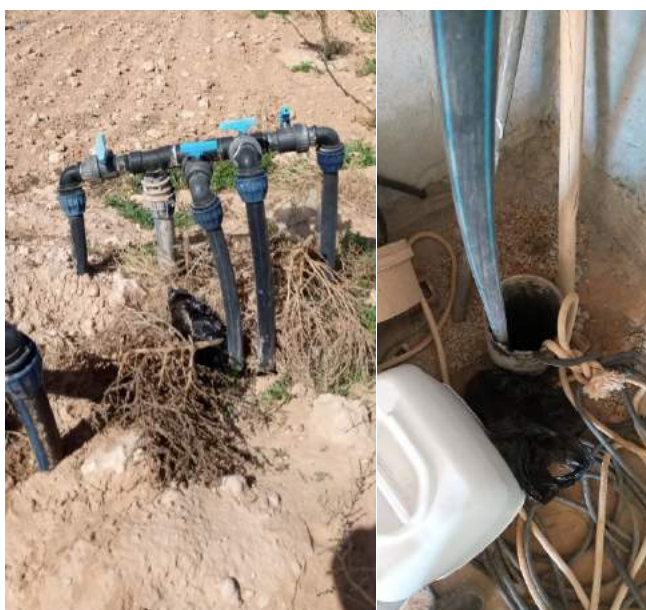
Figure 43: Sounding and irrigation pipes
