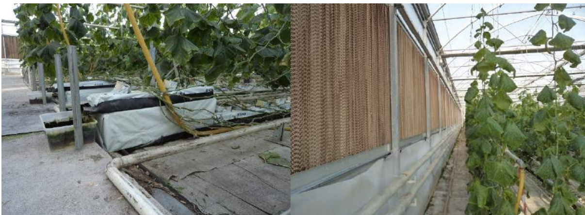
Figure 3. Heating system (floor pipes, grow pipes) and Cooling system (wet pads)
